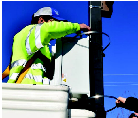
Figure 20: Securing the VLP Communications Box
