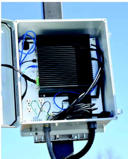
Figure 21: Routing the Power and Camera Cables
